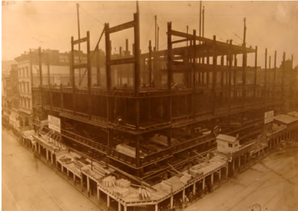
Corner of Washington and Summer streets during erection of the steel frame for the Filene's store, 1912. (source: Filene's Archives, Boston Public Library).
